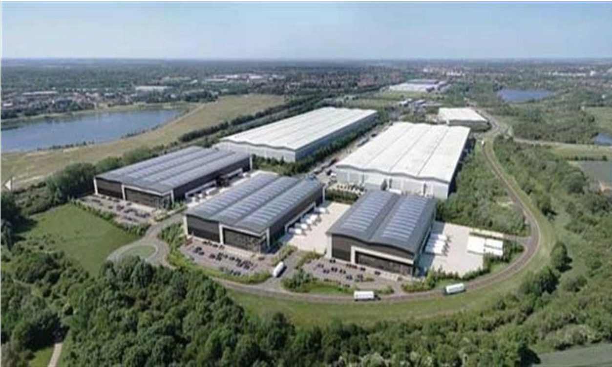
Three Distribution Centres - Kingston Park South, Peterborough
