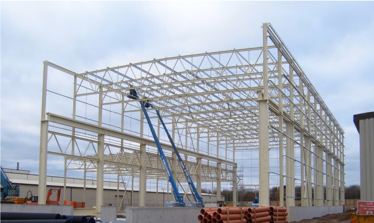
ASCT Building - Honda, Swindon
