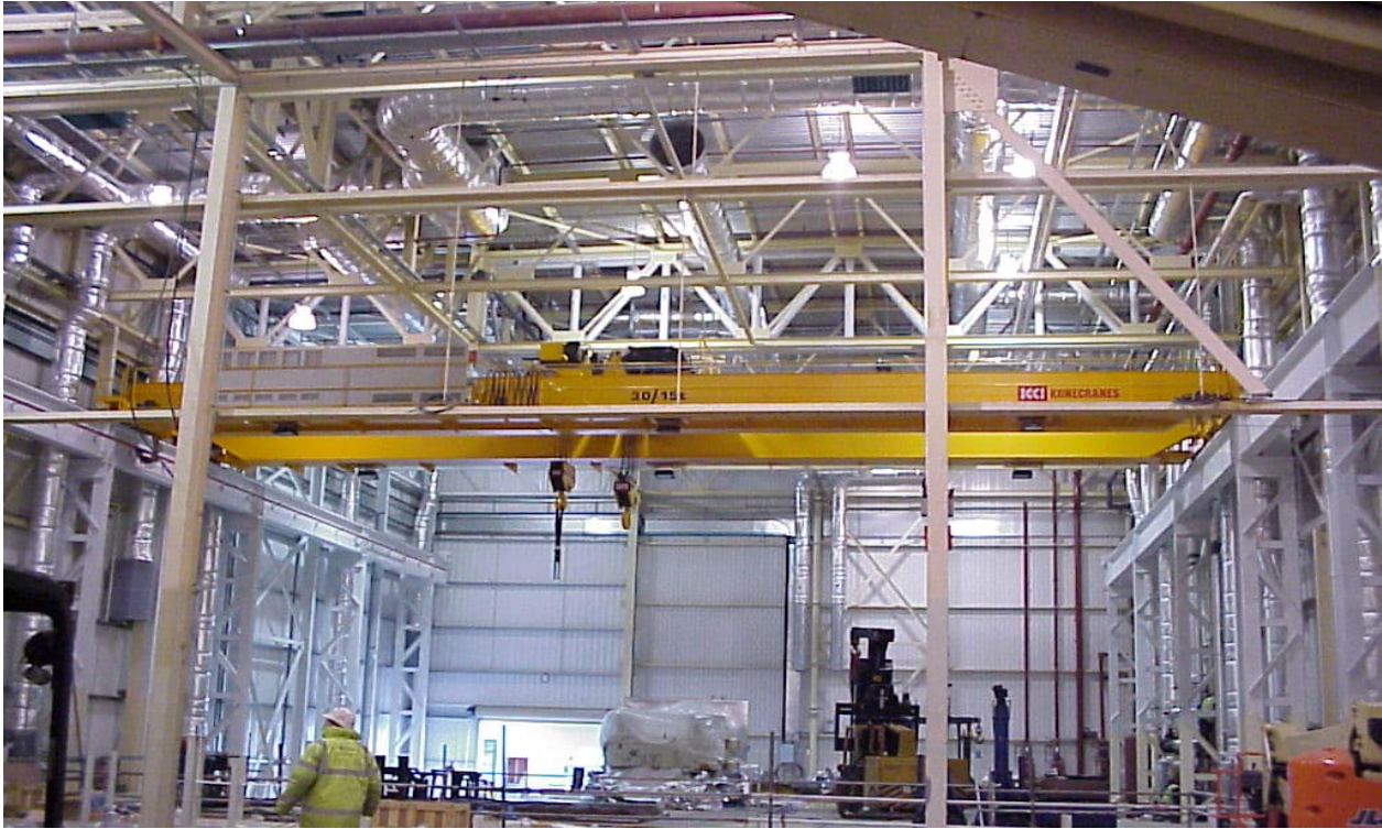
Honda Manufacturing Plant - Swindon
