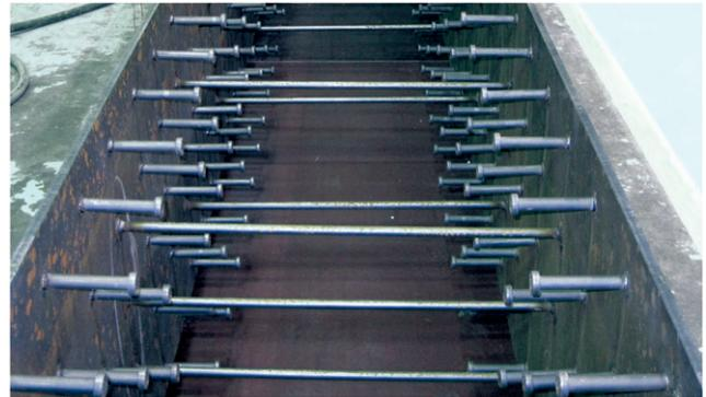
Figure 1. Typical SC panel with bar connectors and shear studs
