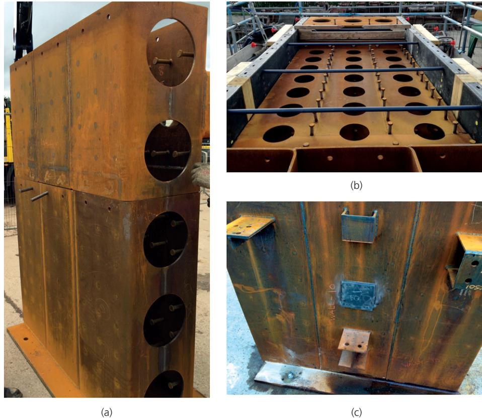
Figure 3. Steel brick (a) walls, (b) floors and (c) attachments
